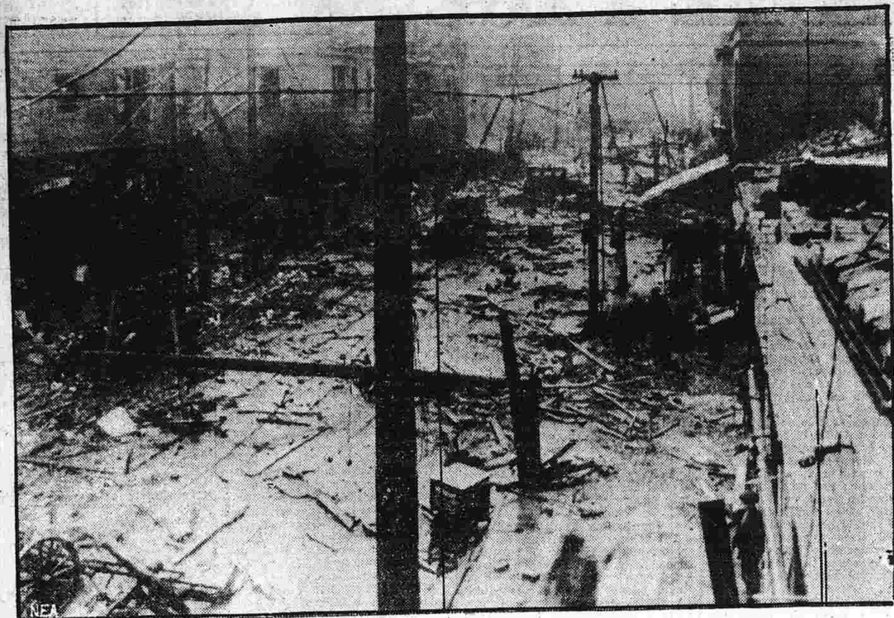
Here is what Enright avenue, St. Louis, looked like after the passage of the cyclone. Note how buildings were ripped apart and the street clogged with wreckage. At the time this picture was taken, immediately after the cyclone had passed on, there were 29 known dead and 100 injured, with more casualties being reported momentarily.
