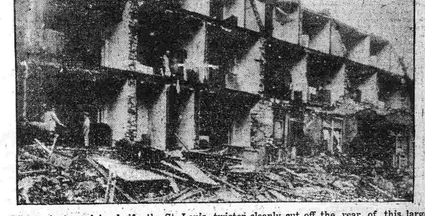
Like a giant revolving knife, the St. Louis twister cleanly cut off the rear of this large apartment house at Maryland Avenue and Whittier Street. Some of the tenants who were not injured may be seen examining what remains of their dwellings.
