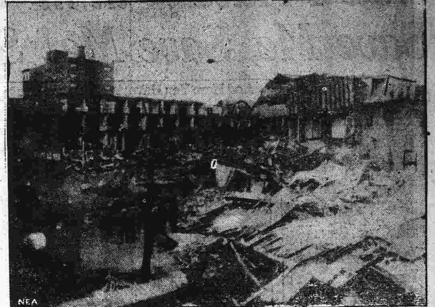
One of the vagaries of the St. Louis twister was to rip away the rear of eight adjoining apartment houses at Maryland avenue and Whittier street, killing or injuring many of the occupants. In this telephoto, rescuers may be seen in the left foreground searching the debris for bodies.
